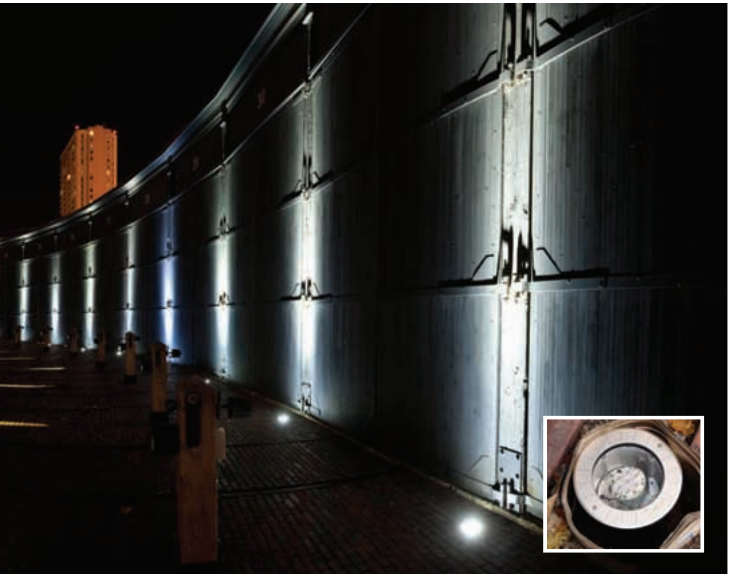
(inset, right) create white stripes on a black building, calling to mind the wheel of a steam train. Meanwhile, the “spokes” of the wheel are created by LED façade and on to the ground.
