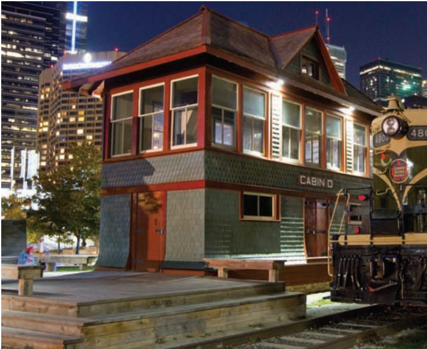
Four and 9-W LED downlights tucked under the soffits of the historic buildings highlight the building features and create illuminated walkways around each one.
